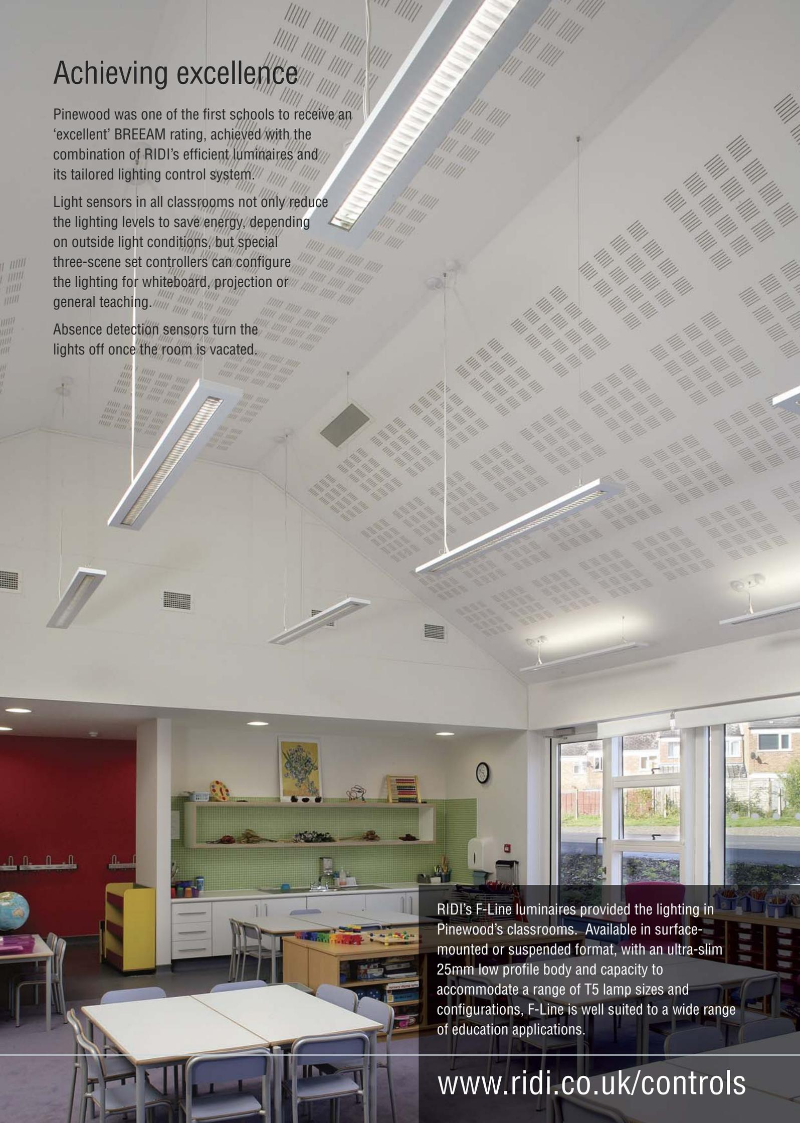
RIDI's F-Line luminaires provided the lighting in Pinewood's classrooms. Available in surface-mounted or suspended format, with an ultra-slim 25mm low profile body and capacity to accommodate a range of T5 lamp sizes and configurations, F-Line is well suited to a wide range of education applications.
